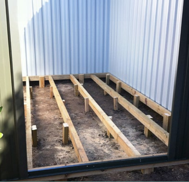
H4 treated timber subfloor
