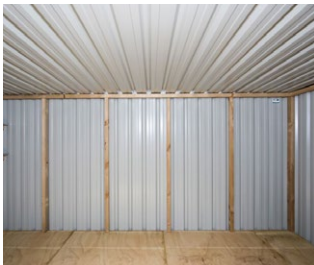
Timber framing gives customers a base to attach shelves, hooks, nails etc.
