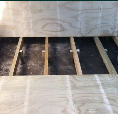
18mm Plywood Flooring
